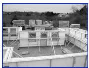
PHOTO BY ROBERT ANDERSEN Called Reddi-Form blocks and made of Styro-Foam, the partially hollow blocks making up this foundation are fitted with steel reinforcement bars and filled with concrete to create super strong walls insulated inside and out to make the house 30 to 70 percent more heat
