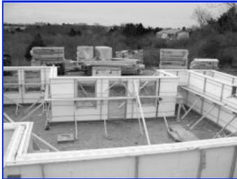
**PHOTO BY ROBERT ANDERSEN** Called Reddi-Form blocks and made of Styro-Foam, the partially hollow blocks making up this foundation are fitted with steel reinforcement bars and filled with concrete to create super strong walls insulated inside and out to make the house 30 to 70 percent more heat efficient.
